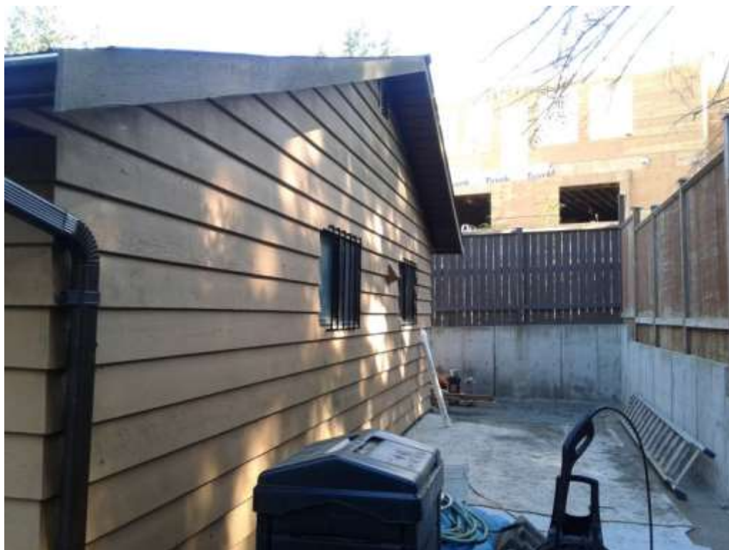
Figure 7: Rear Yard Setback of the Existing Accessory Building
