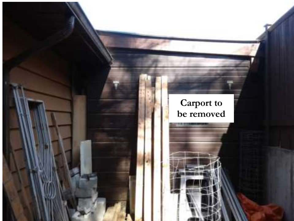
Figure 9: Left (Northeast) Side Yard Setback of the Existing Accessory Building (Note that the carport will be removed.)
